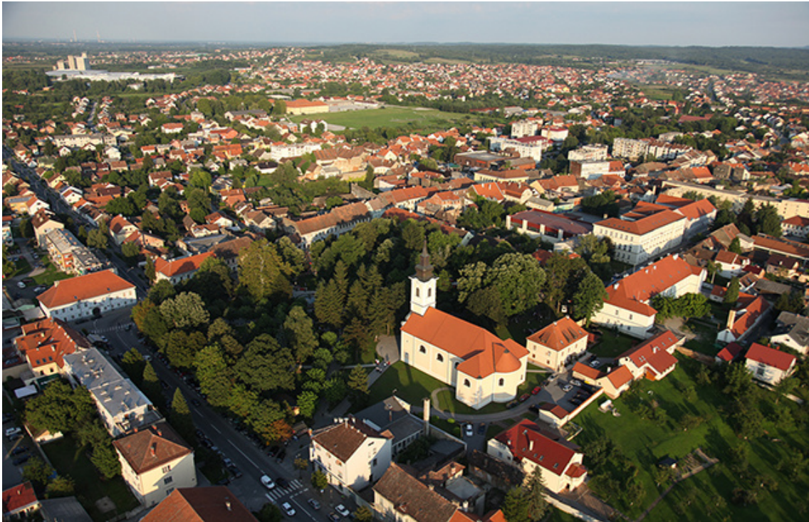
Aerial view on Petrinja's centre
